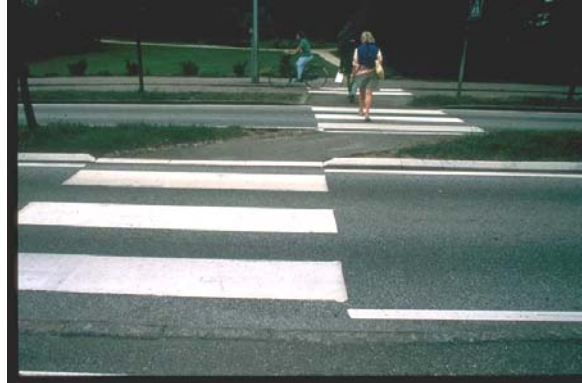
This off-set crosswalk slyly directs cyclists and pedestrians to look in the correct direction before crossing the next section of roadway. This also provides a larger refuge area, which is particularly helpful for cyclists.
