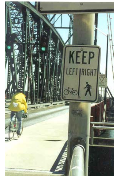
The sidewalks on either side of this Portland, OR metal-decked bridge were widened to become multi-use facilities. There are separate curb-cuts (not shown) for cyclists transitioning from an on-street bike lane and pedestrians continuing from the sidewalk network.
