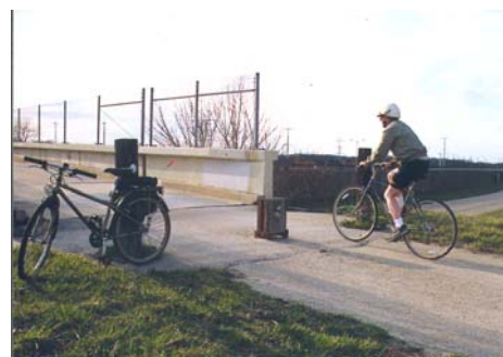
This bollard hinges down to allow a maintenance vehicle to access the bridge. Its placement in the middle of the path allows enough room for cyclists to pass it single file. Reflective paint and a warning sign could help improve its visibility, especially at night. However, if it is unlikely that a motorist would try to access the trail at this location, the bollard could be removed.
