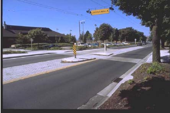
Signage, a center refuge area and push button activated overhead lights increase the visibility of the above mid-block crossing.
